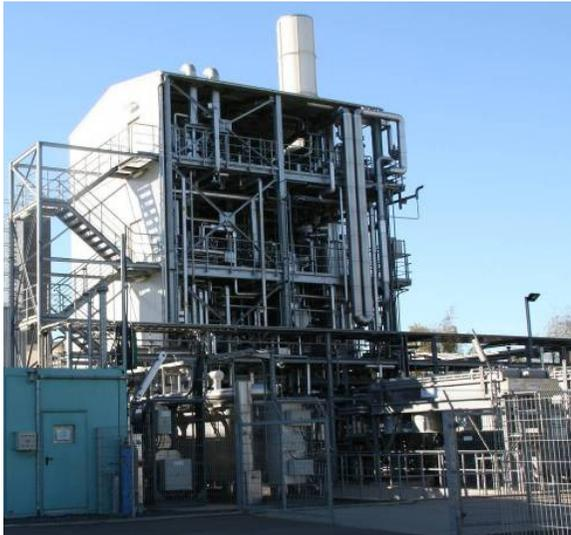
Test plant for high pressure partial oxidation (HP POX) of liquid and gaseous hydrocarbons
