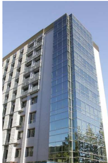
Engineering Research Center
